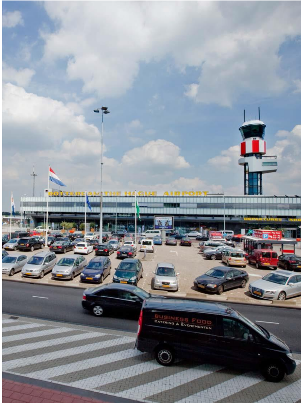
Foto Rotterdam The Hague Airport
