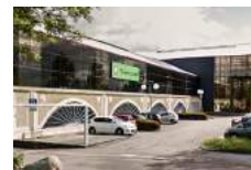
Asphalted parking lot
