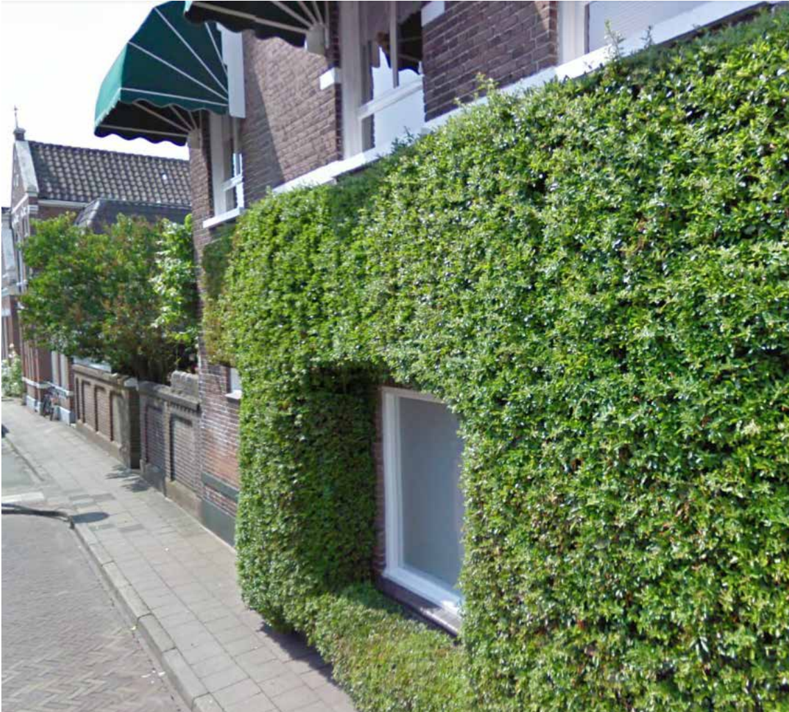
Beplante gevel in Zwolle, Google maps streetview
