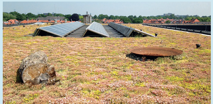
Sedumdak in mei 2018. (Foto: Universal Greenfields)
