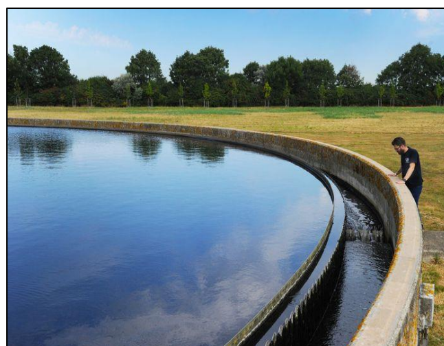
Figure 22, RWZI Kapelle, Retrieved From: https://www.pzc.nl/zeeuws-nieuws/rioolwater-bron-van-de-toekomst~ac7d1431/
