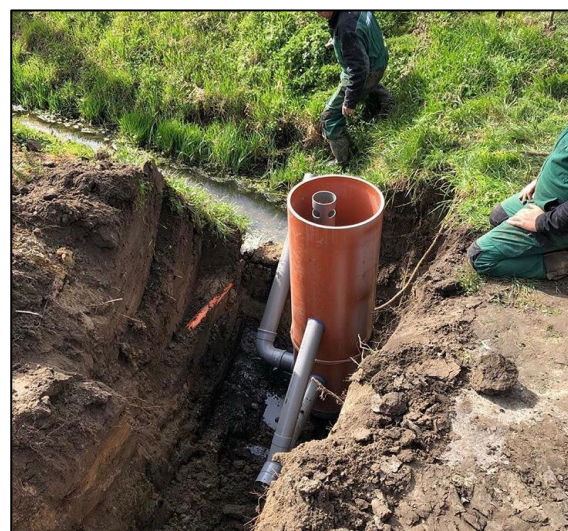
Figure 13, Adjustable Drainage System, Retrieved From: http://www.gebr-emonds.nl/site/drainage/peilgestuurde-drainage.html?showall=1
