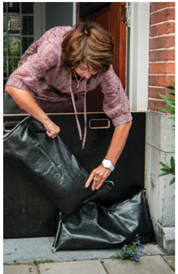
Sand bags and a partition protect against heavy downpours.
