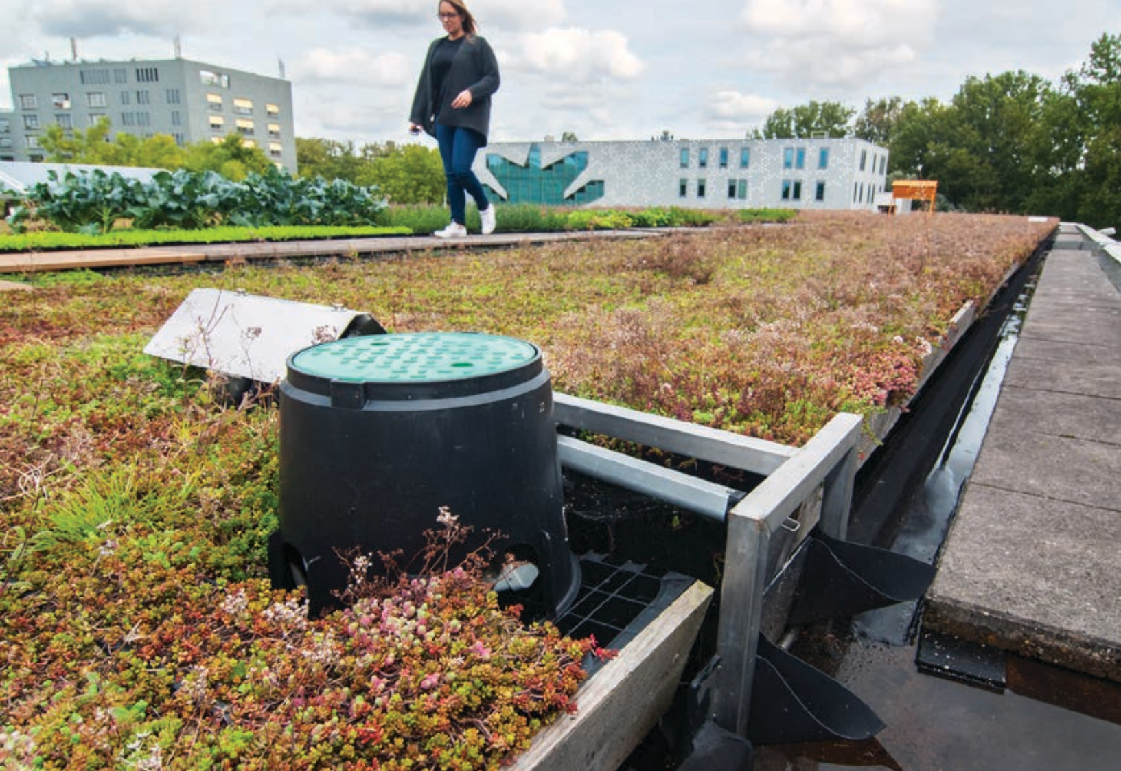
The first polder roof in The Netherlands on top of Old School at Zuidas district.
