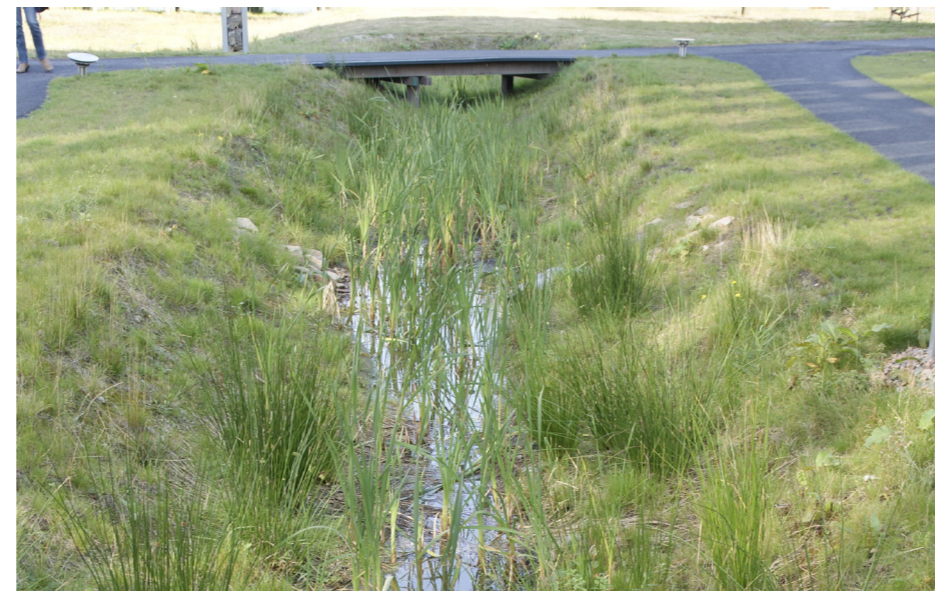
Fig. 11 Infiltratiegreppel, High Tech Campus Eindhoven
